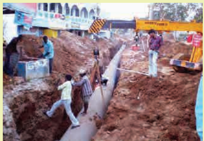
Source: Replacement of Thatipudi pipe line, Andhra Pradesh
